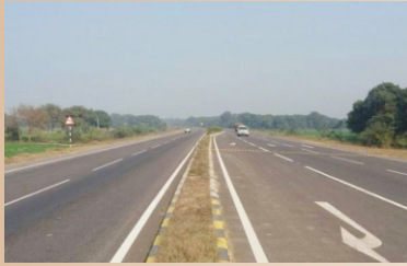
NH 19 PATNA CHHAPRA HIGHWAY
